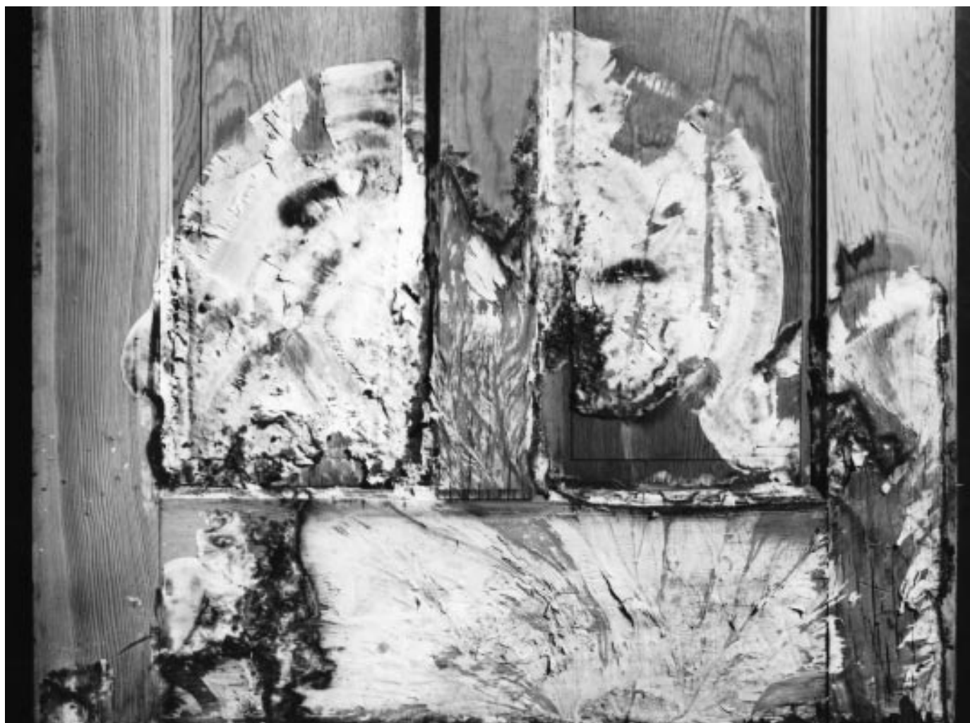
Figure 13–4. Mycelial fans on a wood door.
