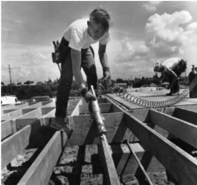
Figure 9-6. A pressurized extruder applies a single bead of elastomeric construction adhesive to floor joists for assembly of a plywood floor system.
