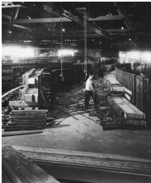
Figure 11–5. After being placed in the clamping bed, the laminations of these arches are forced together with an air-driven screw clamp.
