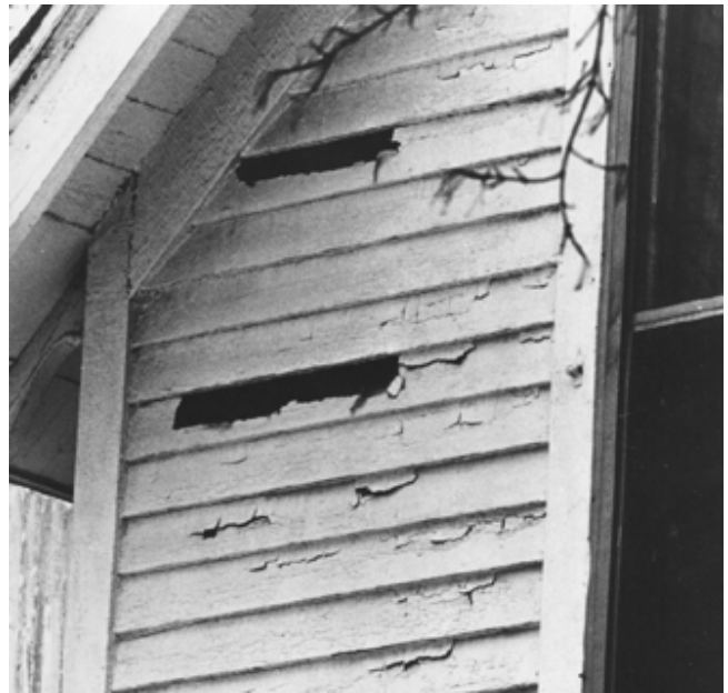
Figure 15–15. Paint can peel from wood when excessive moisture moves through house wall. Some cross-grain cracking is also evident on this older home.
