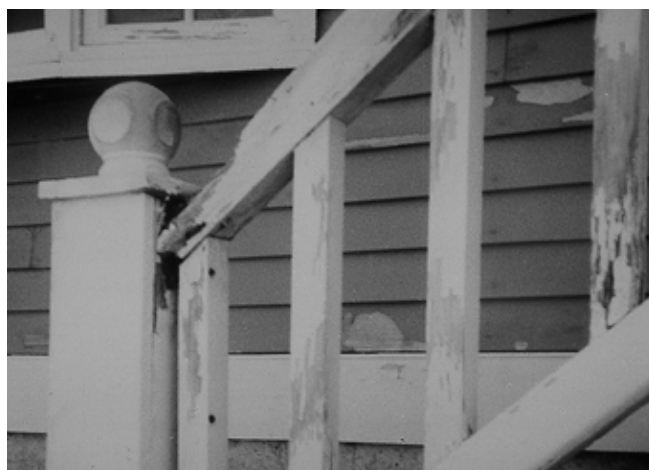
Figure 15-10. Decay in wood railing fully exposed to weather.
