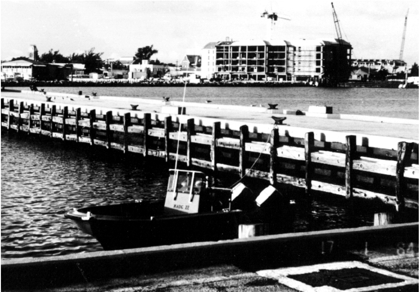
Figure 1–2. Wood is favored for waterfront structures, particularly fendering, because of its shock-absorbing qualities. The fendering on this dock in Key West, FL, is made of creosote-treated Douglas-fir ( Pseudotsuga menziesii ). Some tropical species are resistant to attack by decay fungi and marine borers and are used for marine construction without preservative treatment.
